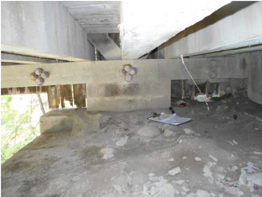
Existing Bearing Blocks
