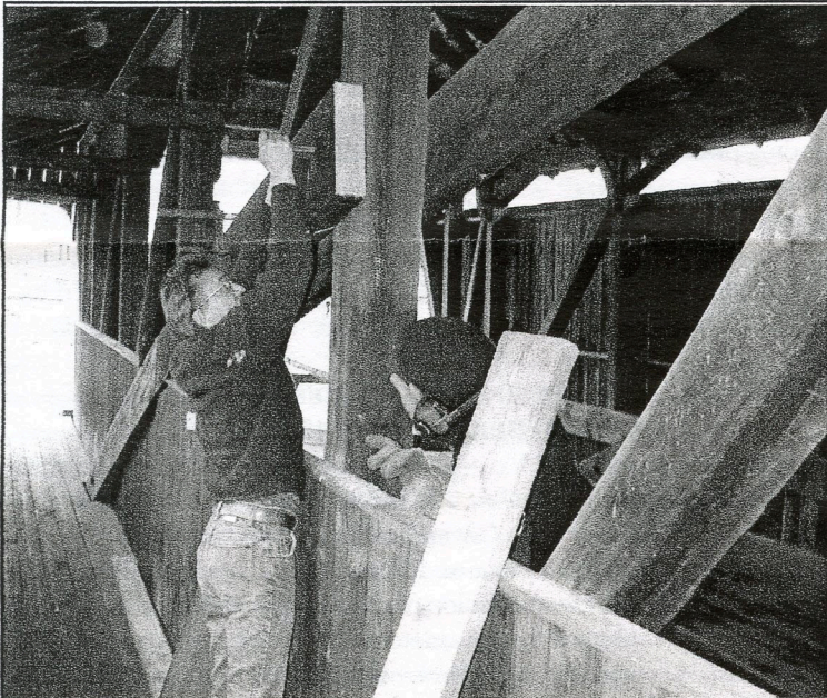
Jan Lewandoski (right) and Mike Cotroneo remove broken Burr-arch segment from the Waitsfield Village Bridge. Photo by Joe Nelson
