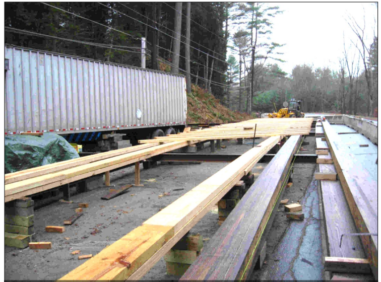
Williamsville Bridge construction site - lattice construction w/ bottom chord Glulam, by Ray Hitchcock November 2009
