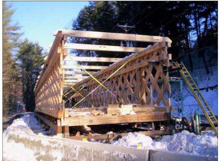
**January 19, 2010** - We stood up the second truss today and installed tie rods underneath and tie beams overhead - Photo by Jim Ligon
