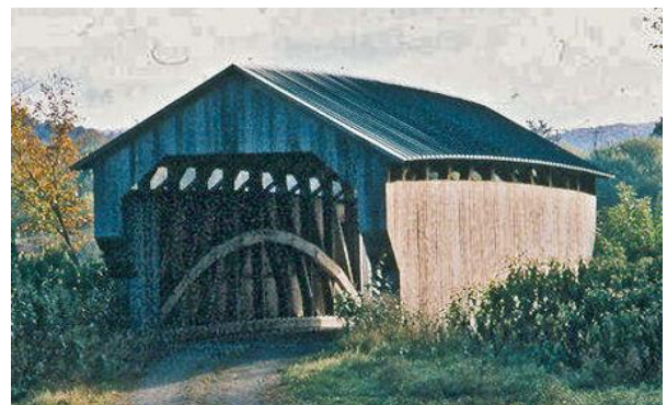
Gates Farm Bridge, Photo by Joe Nelson, Summer 1997
