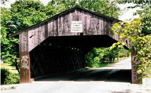
Maple Street Bridge, Photo by Joe Nelson, Summer 1995
