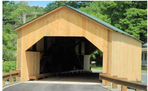
East Fairfield Bridge, Photo by Joe Nelson, summer 2009
