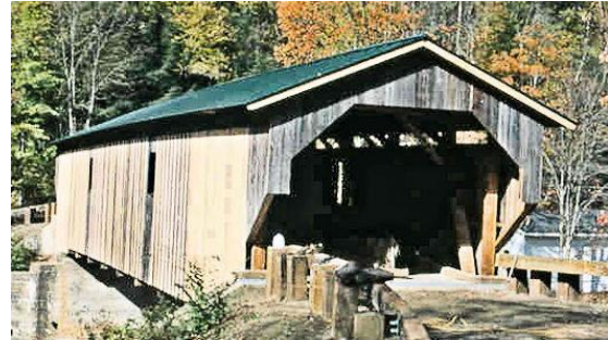
Grist Mill Bridge, Photo by Joe Nelson, October 2004
