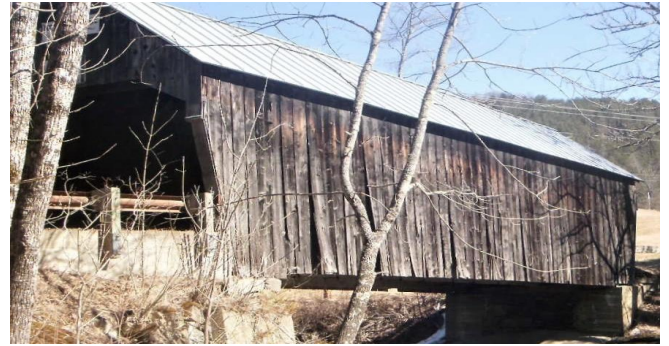
Moxley Bridge, Photo by John Weaver
