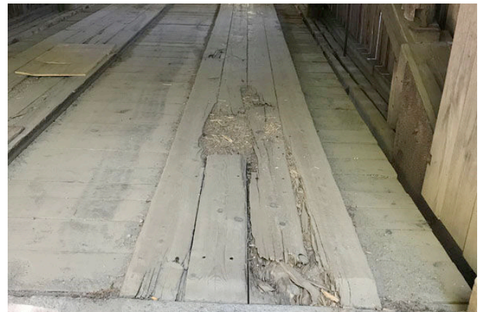
Morgan Bridge, photo by Steve Miyamoto, June 2020
