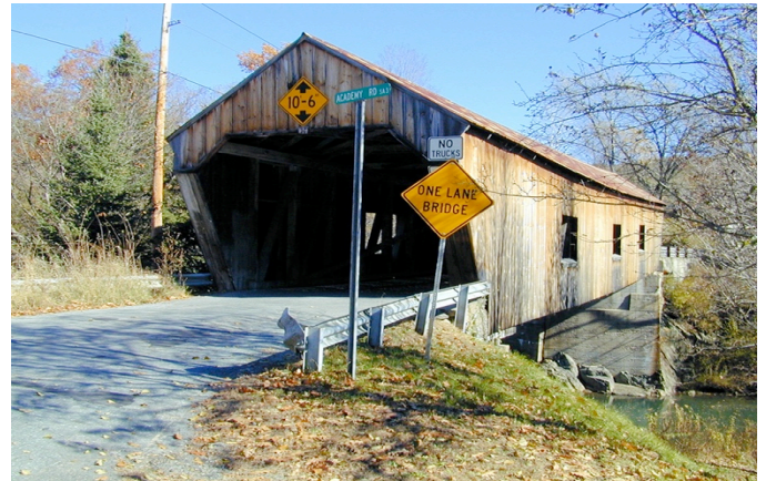
Union Village Bridge, photo by Joe Nelson, June 2014
