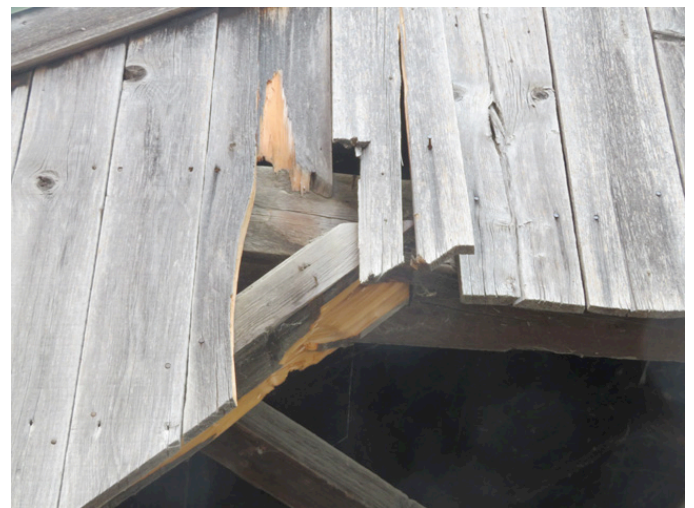
Kingsley Covered Bridge, photo by Edwin Loveland
