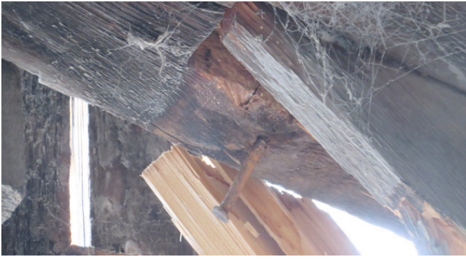
Kingsley Covered Bridge, photo by Edwin Loveland
