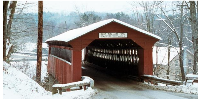
Chiselville Bridge, photo by Joe Nelson, 1997
