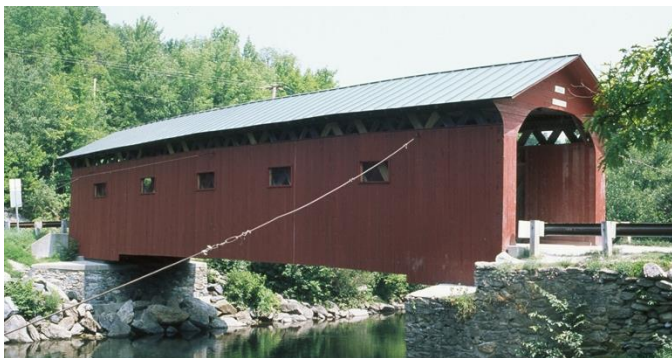
Bridge-at-the-Green, photo by Joe Nelson, 1997
