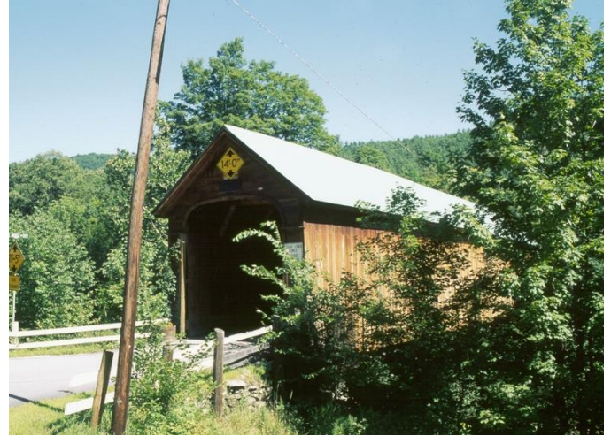
Hall Bridge, photo by Joe Nelson, 1997
