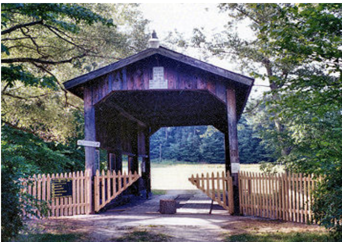
Mill's Riverside Park Bridge [45-04-B], submitted by Joe Nelson
