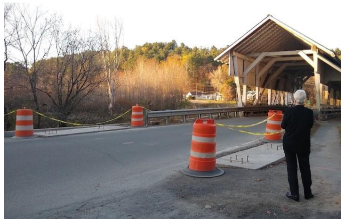
Jeanne Beaudry surveying new footings for steel beams at Millers Run CB - photo by Marcel Beaudry
