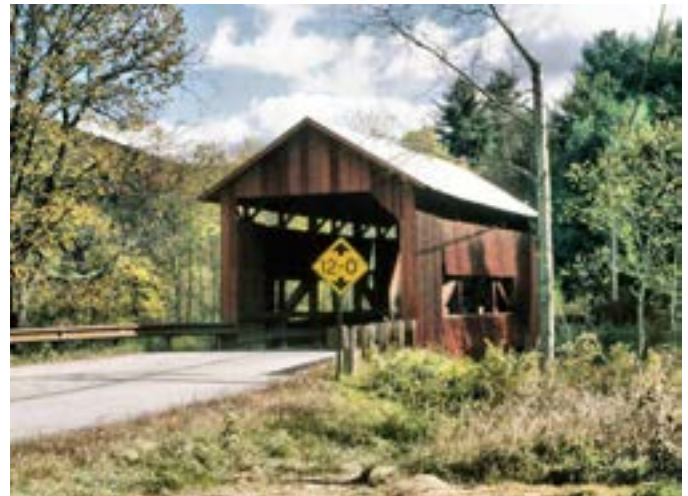
Upper Cox Brook Bridge, Photo by Joe Nelson, 1997
