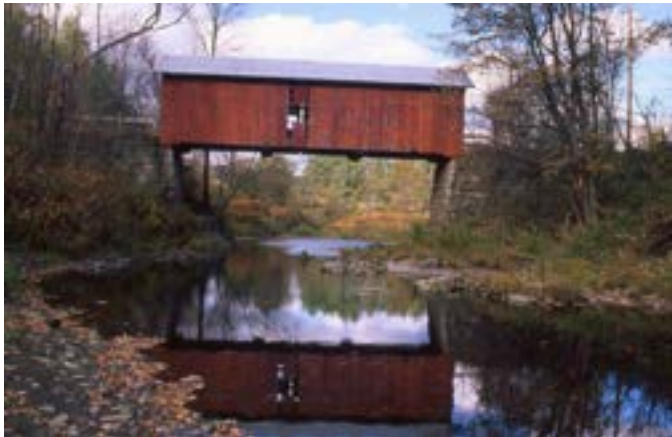
Slaughter House Bridge, Photo by Joe Nelson, 1997
