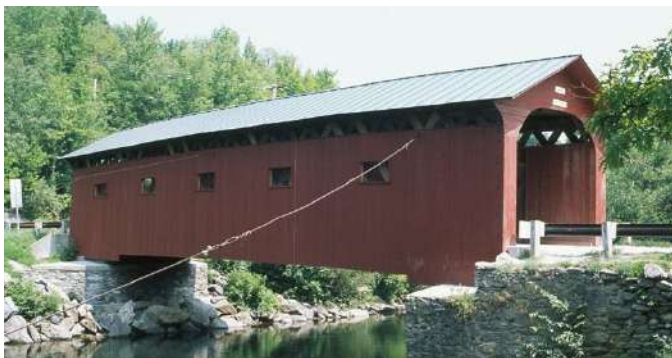
Bridge-at-the-Green, photo by Joe Nelson, 1997
