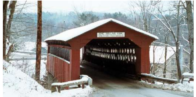
Chiselville Bridge, photo by Joe Nelson, 1997
