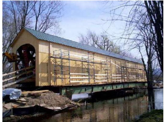
Salisbury Station Bridge, Good for the next 100 years photo by Joe Nelson, April 23, 2008
