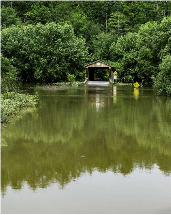
Gorham Covered Bridge, Pittsford Photo by Peter Cosgrove, July 2023
