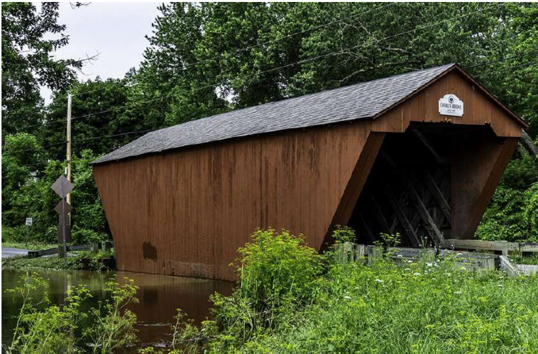
Cooley Covered Bridge, Pittsford Photo by Peter Cosgrove, July 2023
