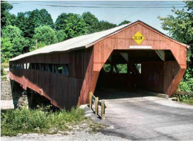
Taftsville Bridge, photo by Joe Nelson, 1997
