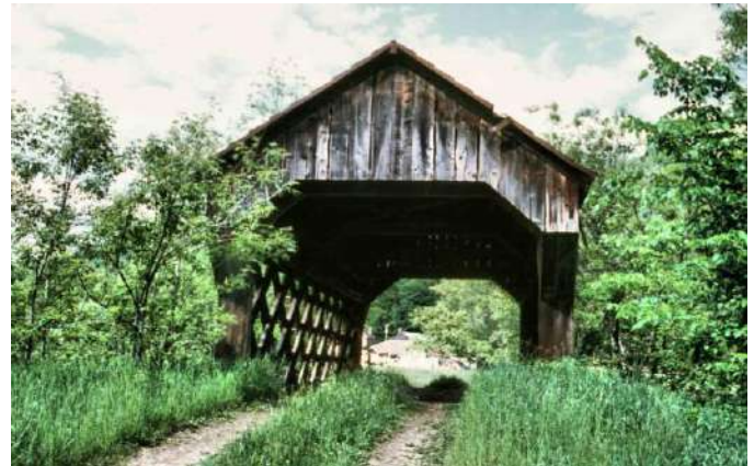
Smith Bridge at Pomfret, photo by Joe Nelson, 1997
