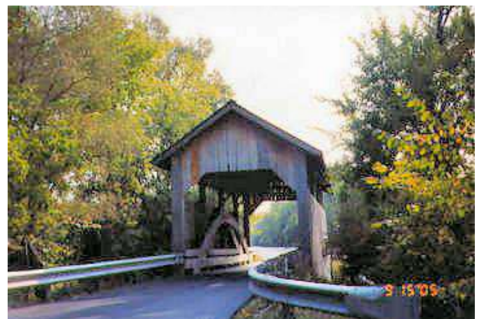
Lakeshore Bridge, photo by Tom Keating, September 2005
