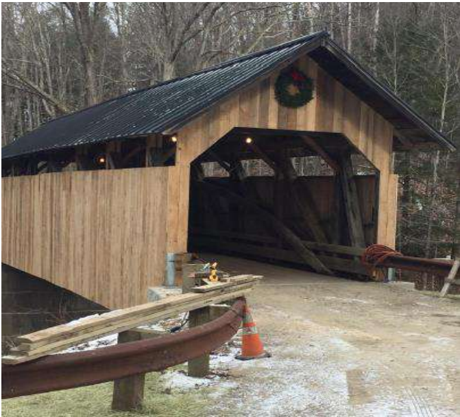
Seguin Bridge, photo courtesy of VTrans
