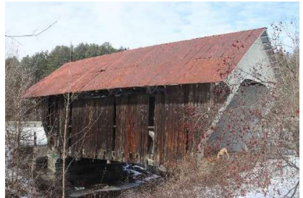
Winston inspecting the Schoolhouse Covered Bridge – by Mark Maddox
