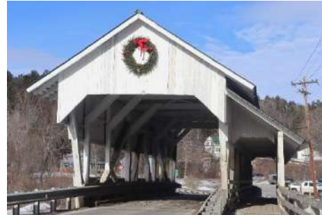
Millers Run Bridge 5 days prior to accident – by Mark Maddox
