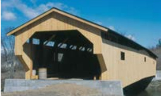
Cambridge Junction Bridge, Photo by Joe Nelson, Summer 2004
