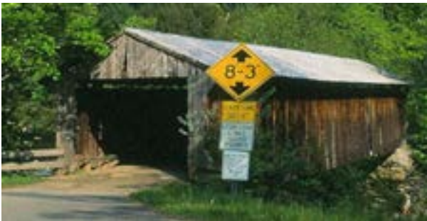
Montgomery Bridge, Photo by Joe Nelson, summer 1995
