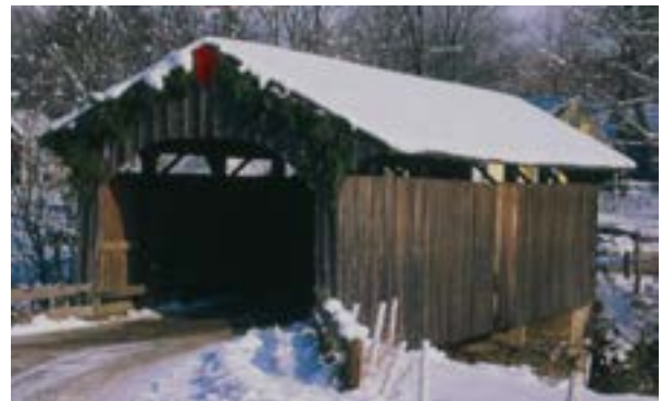
Church Street Bridge, Photo by Joe Nelson, winter 1995
