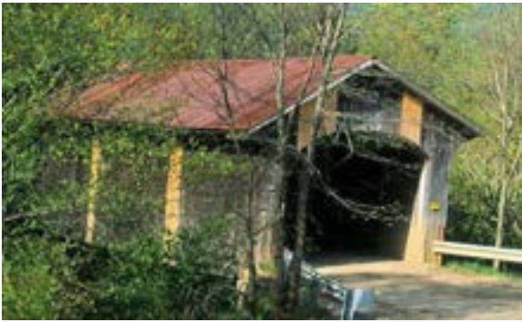
Lumber Mill Bridge, Photo by Joe Nelson, summer 1995
