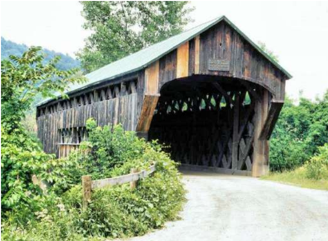
Worrall Bridge, photo by Joe Nelson, 1997
