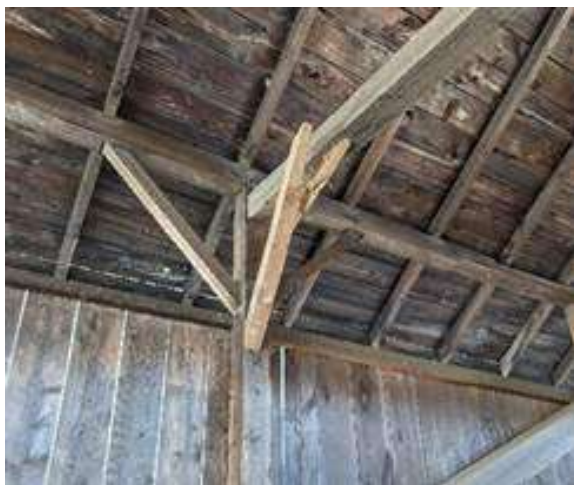
Village or Church Street Bridge
