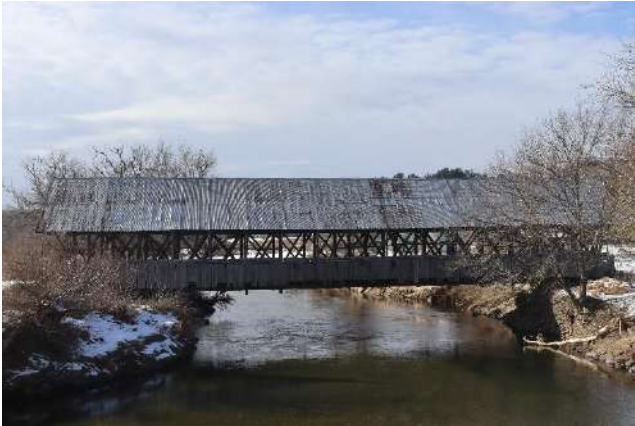
Sanborn Covered Bridge prior to being disassembled - photo by Mark Maddox
