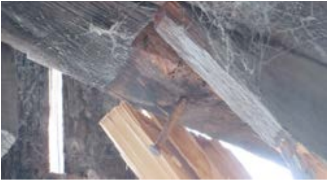
Kingsley Covered Bridge, photo by Edwin Loveland
