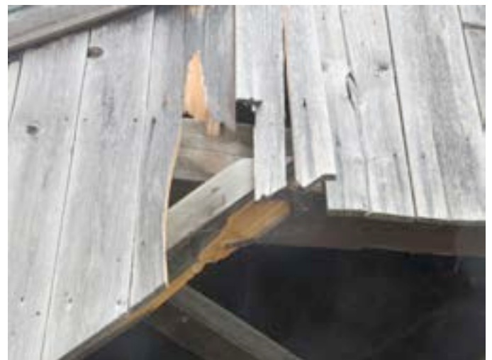
Kingsley Covered Bridge, photo by Edwin Loveland
