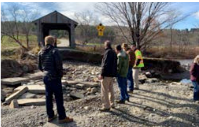
Scribner Covered Bridge, photo courtesy Governor's Office
