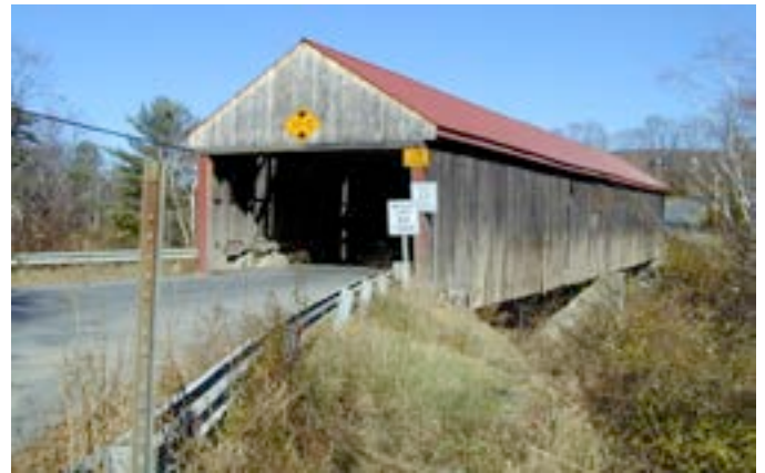
Sayres Bridge, photo by Joe Nelson, June 2014
