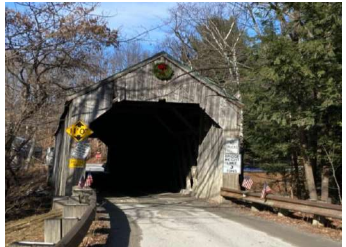
Kingsley Covered Bridge, Photo by Beth Brown-Limmer
